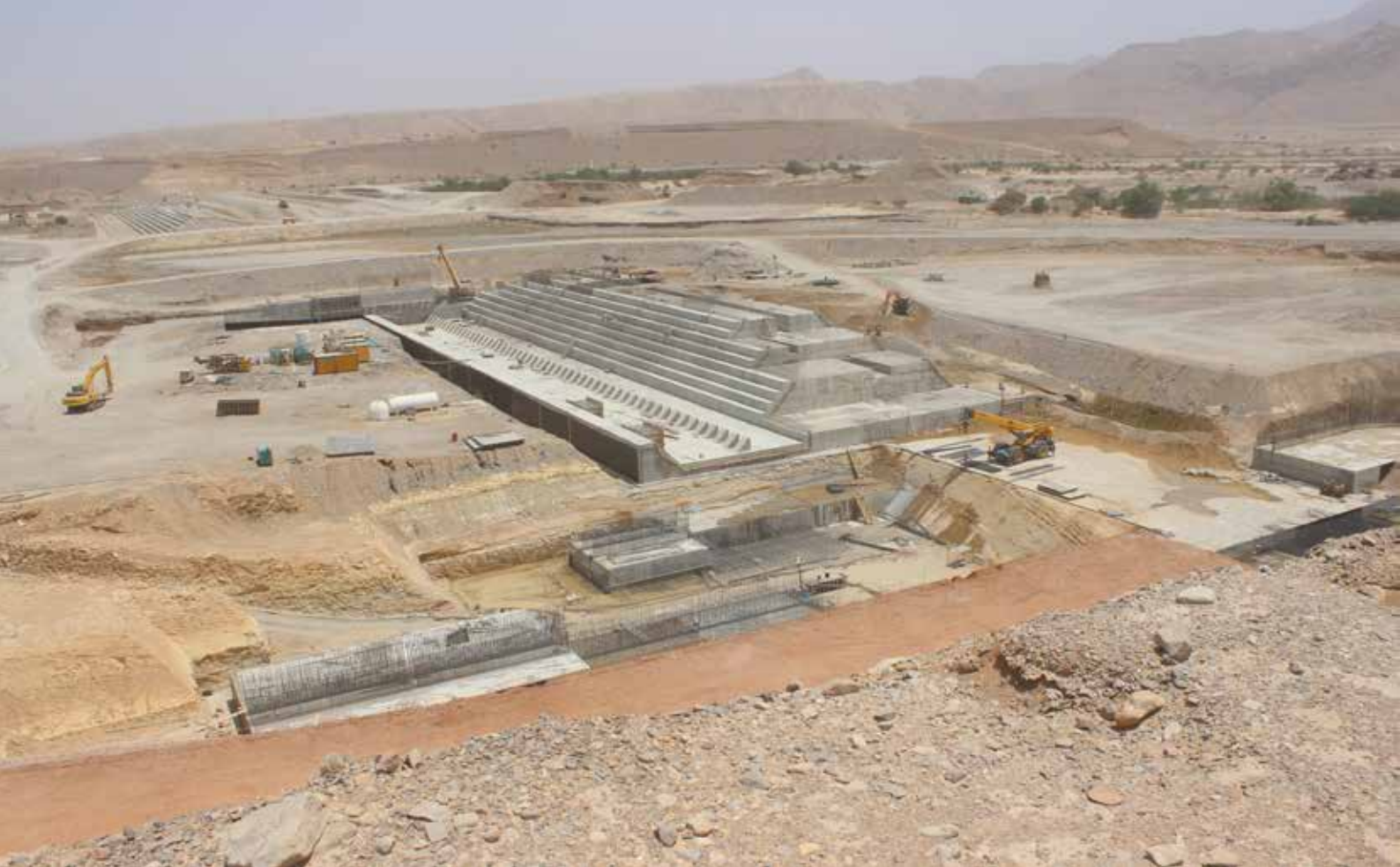
Construction of the spillway © STRABAG International GmbH
