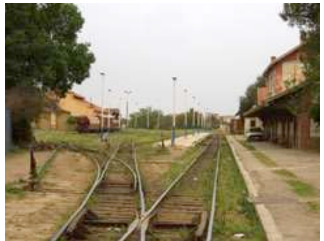
Existing buildings at Saida Station
