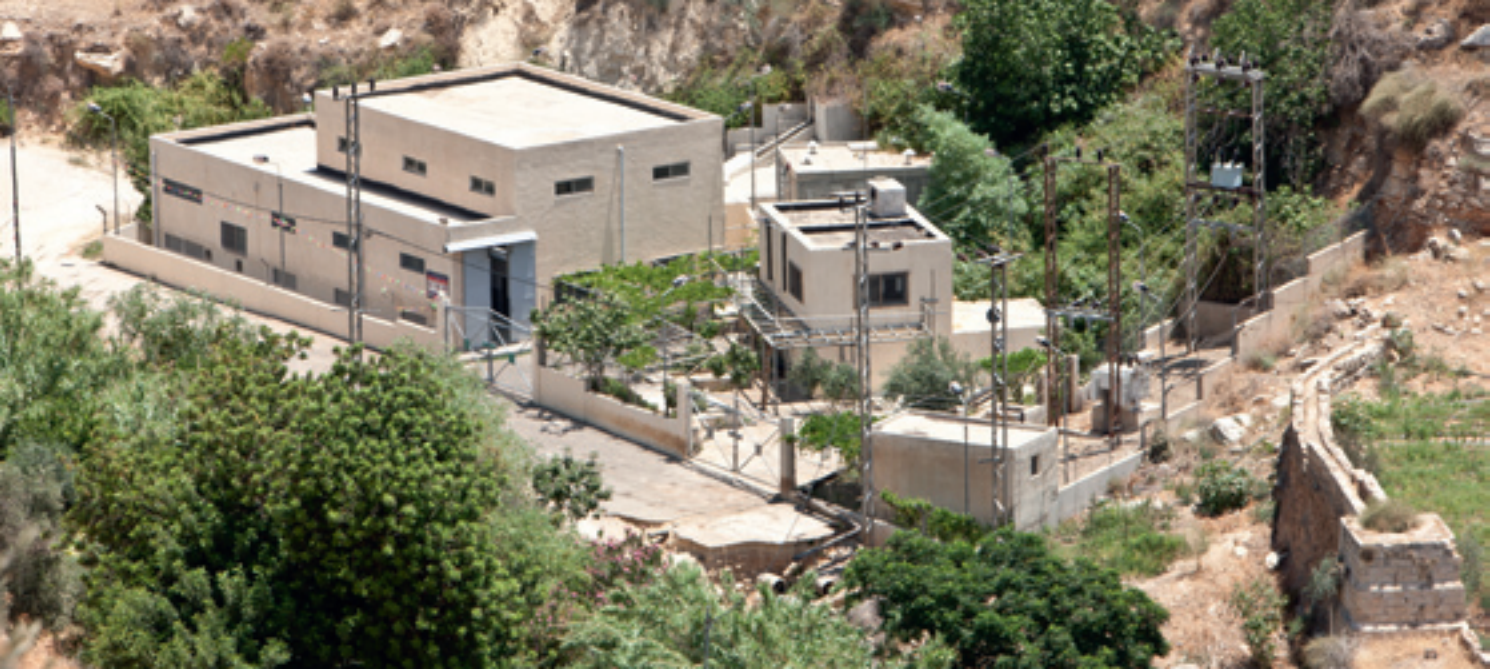
Water Pumping Station (Picture courtesy of WJLO SE)
