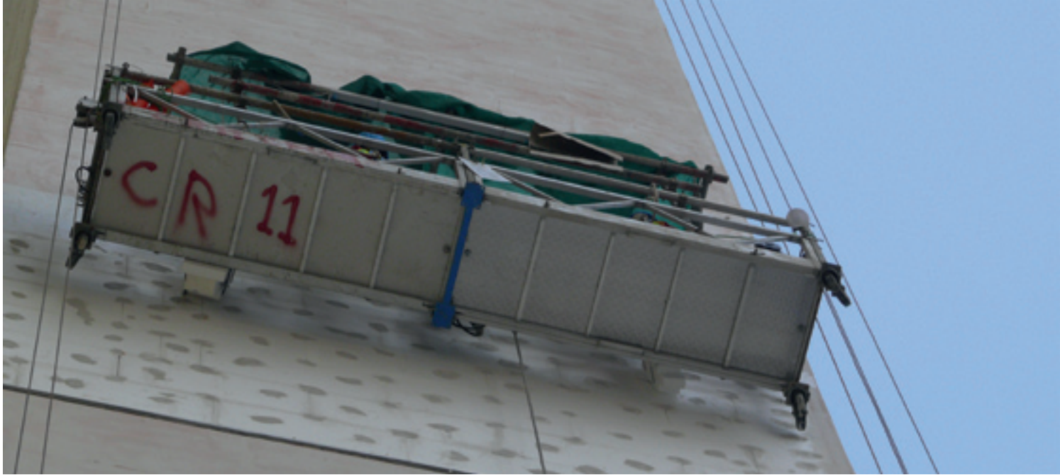
The suspended “cradle” used for the ETICS installation
