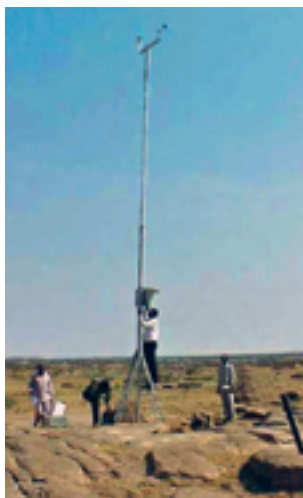
Installation of a wind measurement station in Nyala in 2001
