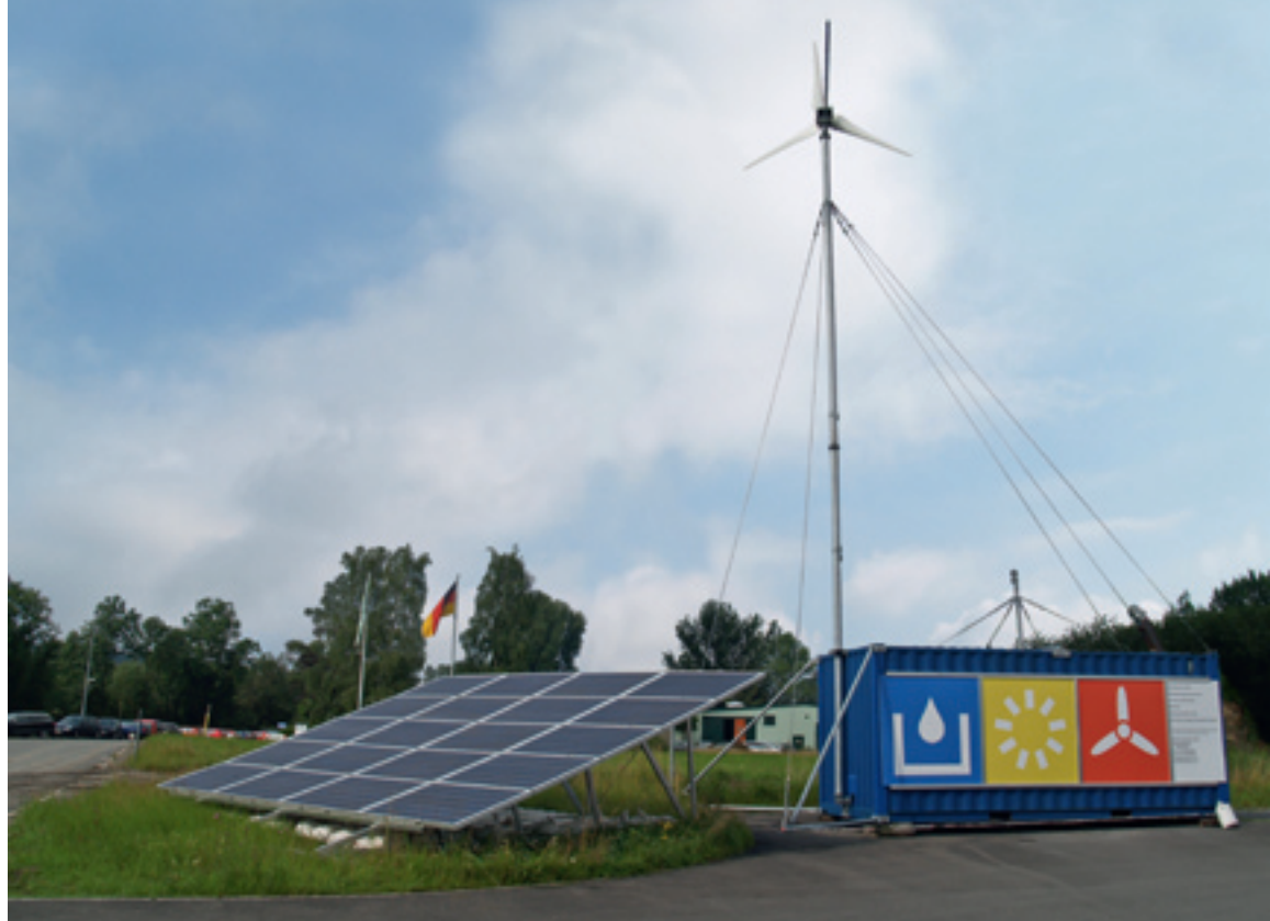
“Power&Life Container” installed in Neuenrade, Germany.
