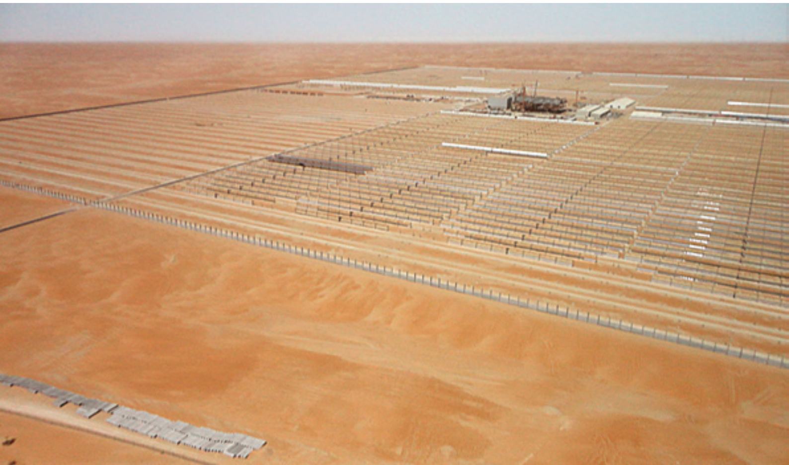
Shams One Plant construction site
