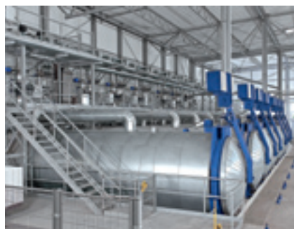
Autoclaves for optimised curing
