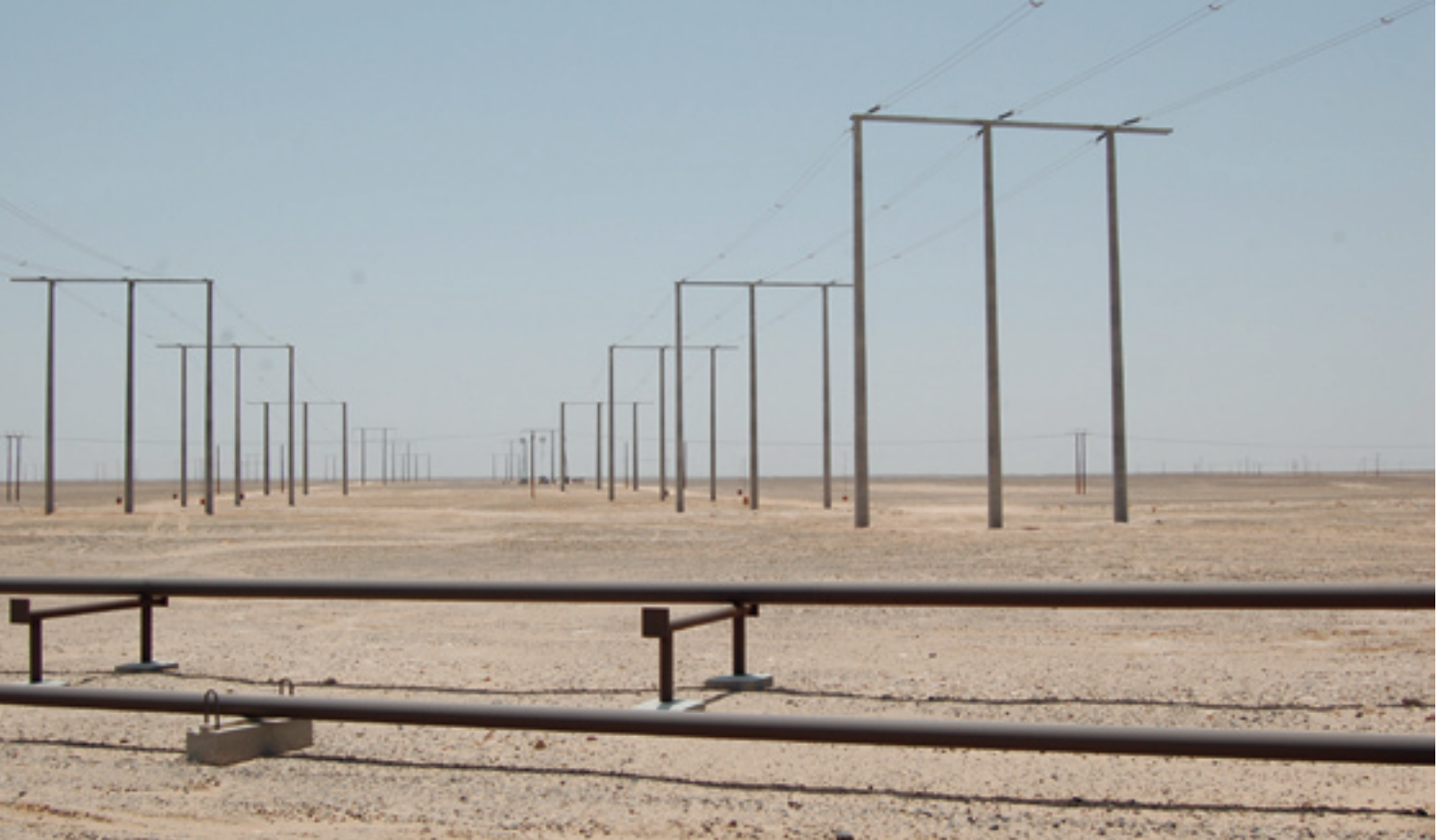
Installation of a 132 kV line on concrete masts, near Nimr, in Oman
