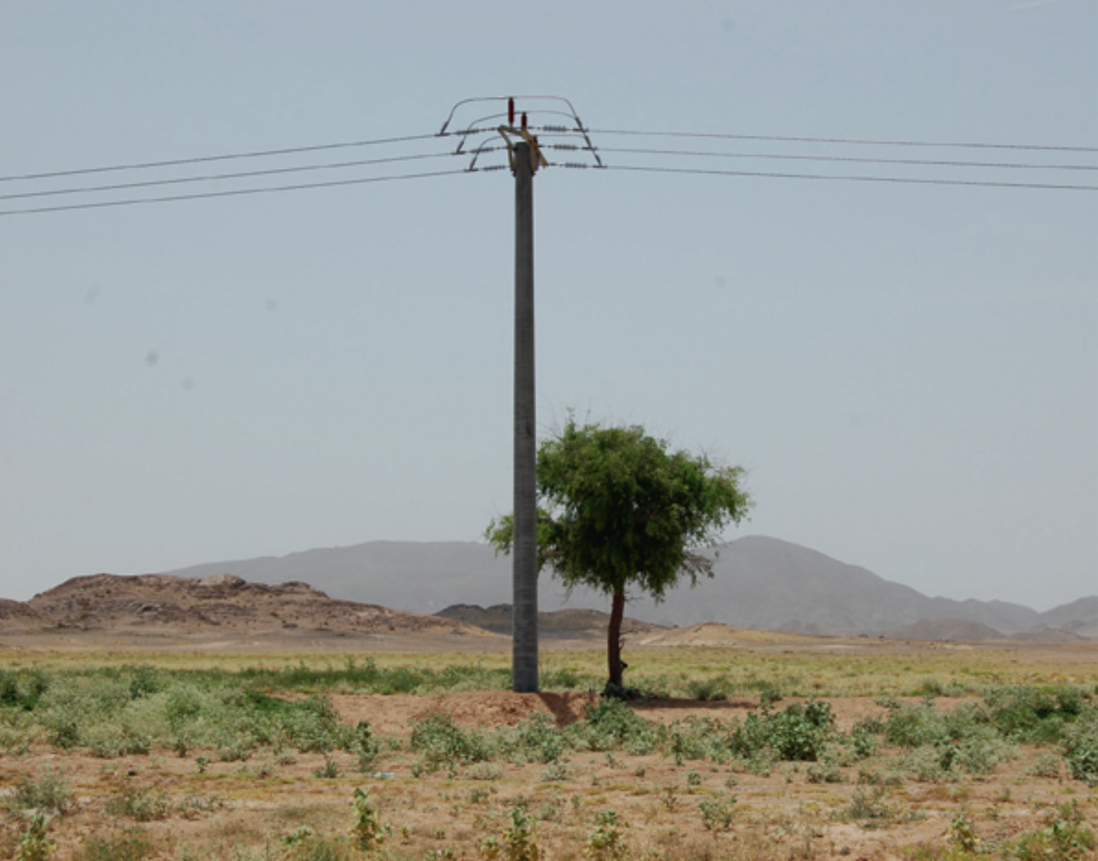
A 33 kV section pole in a coastal area, near Al Ashkara, Oman
