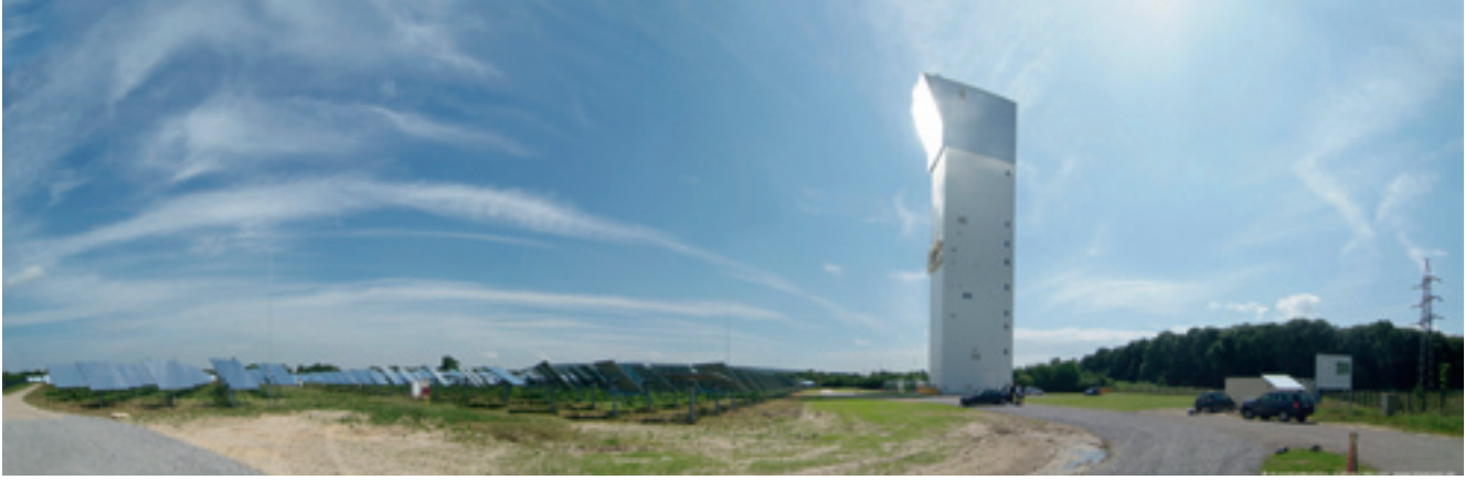
Solar investigation tower in Jülich, Germany
