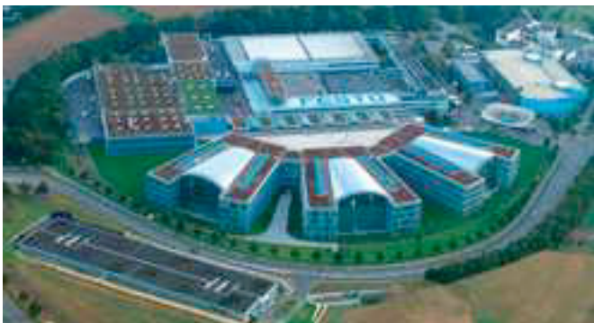
1 | Festo AG & Co. KG headquarters in Berkheim, Germany
